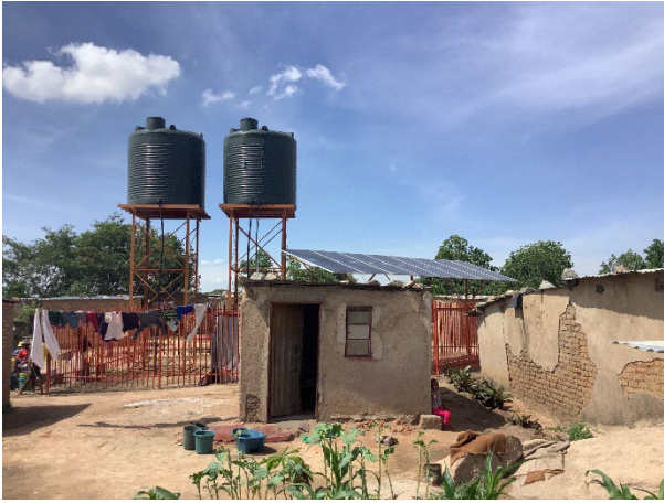
Figure 7-5: Community Borehole in Zone 5 Hopley
