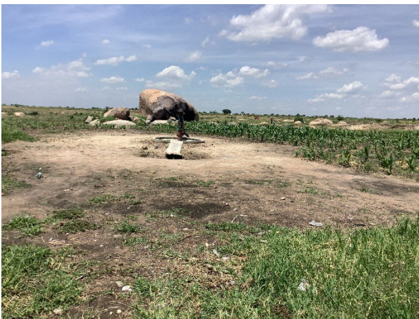
Figure 7-7: Non-functional community bush pump Source: Fieldwork, December 2024
