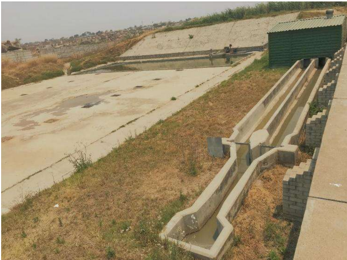
Figure 7.132: Constructed Treatment Plant in Stoneridge
