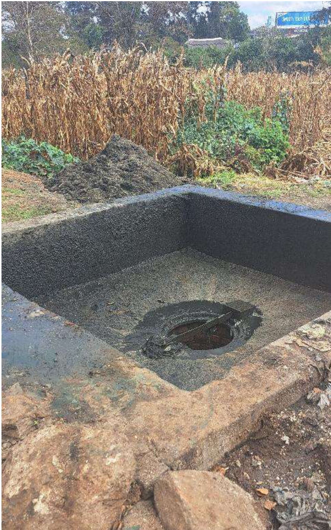
Figure 7.130: Open Outfall Manhole Newlands
